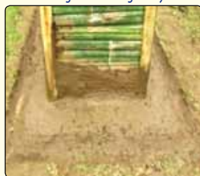
Construction of moat around the tank
