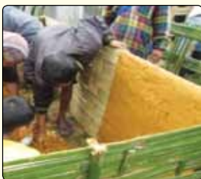
Plastering of the inner walls of the tank
